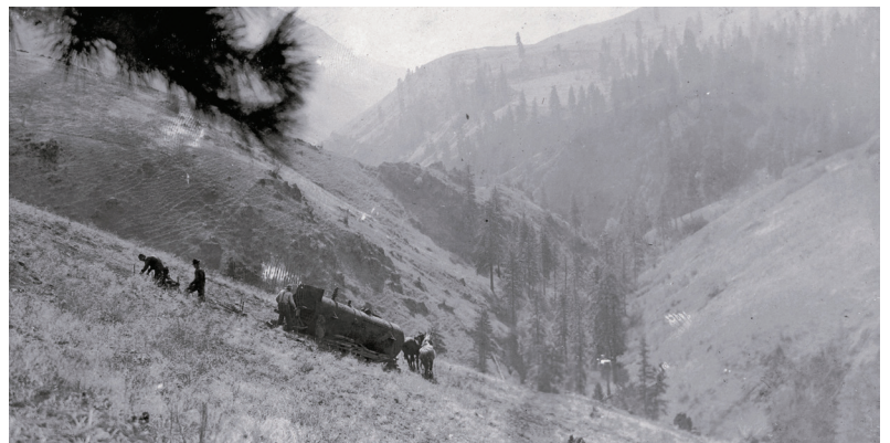
Transporting equipment to the Mill at Deer Creek Mining & Milling Co
